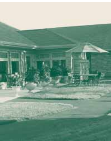
The Stabler Centre Hospice Niagara
